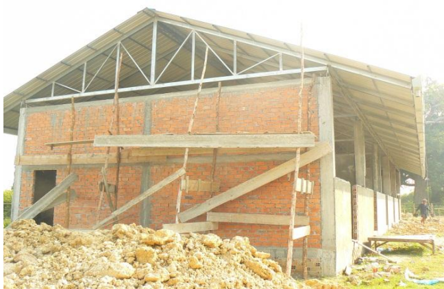
(This is the third building for child day care service)
