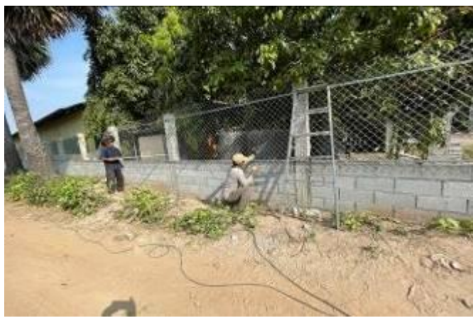
Metal & Brick Fence Construction Project
